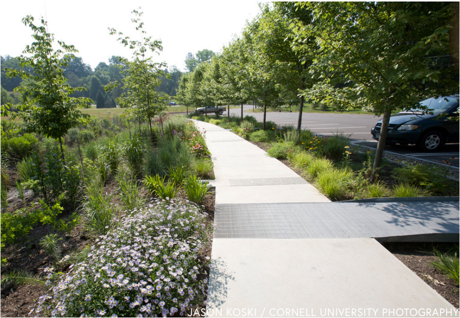
This sidewalk allows water to flow underneath. Water is then filtered by native vegetation before entering waterways.
