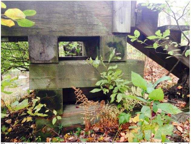
Photo 10: View of crib pier supporting bridge—may not be necessary for proposed Torrey Brook bridge.
