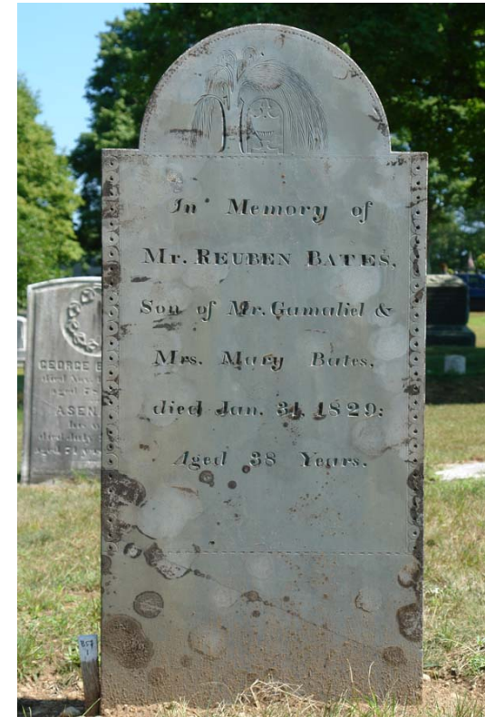
B. 57.1 Rueben Bates Before and after— severely tilted . Early slates and marbles were often set as deeply in the ground as what appeared above the ground.
