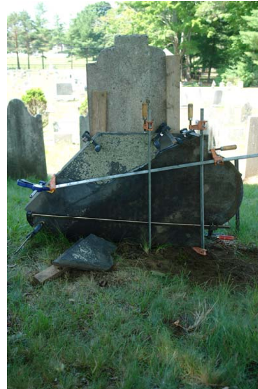
Clamping and bracing in a vertical position allows gravity to help position fragments.
