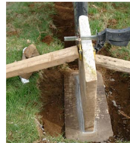
Lower fragment of fractured marker first reset into slot and braced. Top fragment will be attached with structural adhesive after grout has sufficiently cured.
