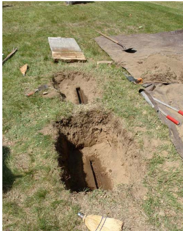
Original bases were raised to an appropriate level, aligned with adjacent markers and set plumb before resetting the markers.
