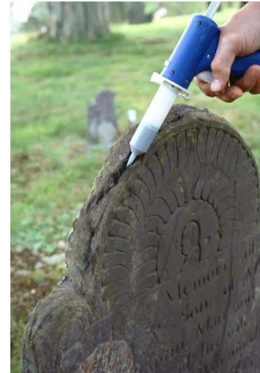
Filling top cavities with a pigmented crack filler by Sto. Material can be applied by trowel or injection. Excess material is immediately wiped off with damp sponging
