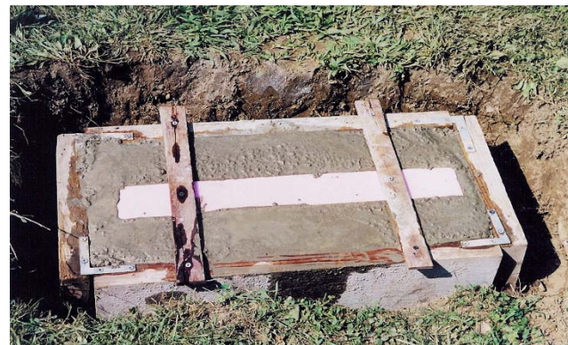
Concrete poured, with form for setting slot in place
