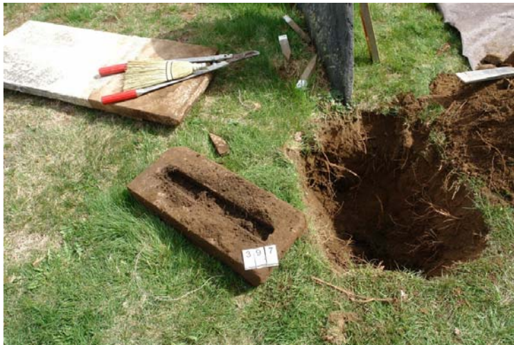
When excavating for resetting often original, or old bases are discovered
