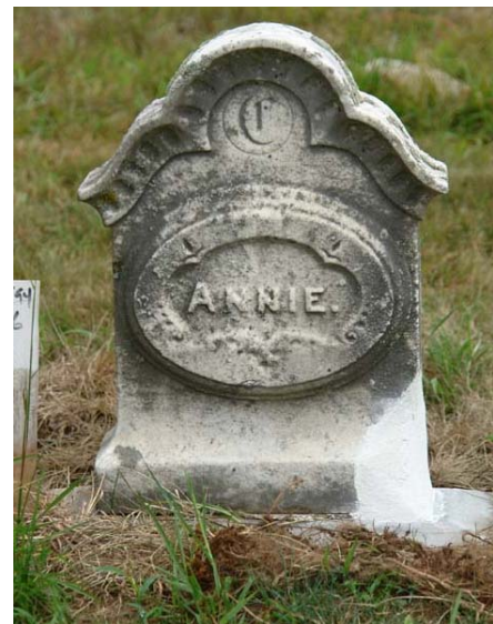
#E94.6 Annie Chamberlin with loss filled with Jahn M70 mortar
