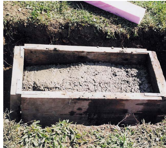
Form for new below grade concrete base
