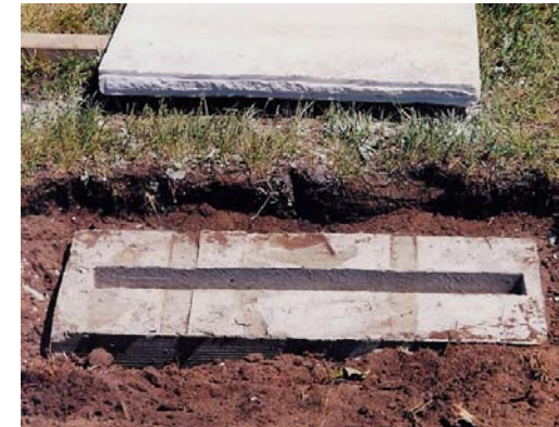
Form removed, ready for resetting marker
