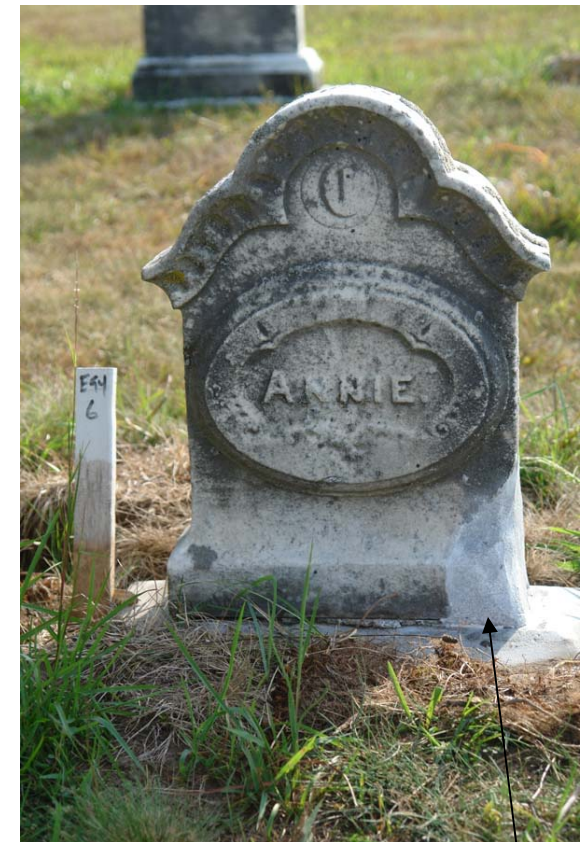
Jahn M70 mortar patch, with artificial weathering
