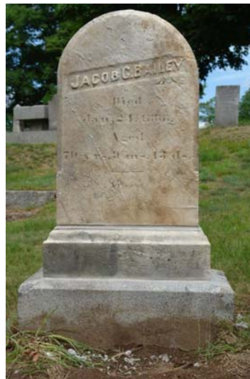
D20 Jacob Bailey reset onto existing base.
