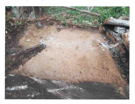
**8.)** Excavation test pit to sixteen (16) feet below grade, between concrete pad # 4 and # 5 virgin granular gravel and sand evidence of debris, residuals of magnesium, no PID readings, petrolem / hazardous materials stains olfactory odors. Note: Sampled for magnesium and 8 RCRA metals.
