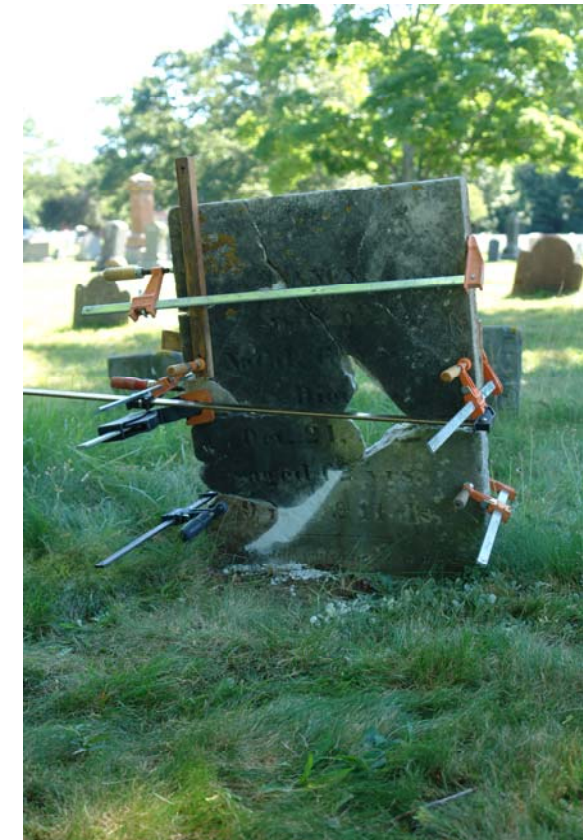
Clamping and bracing in a vertical position allows gravity to help position fragments. Often marble becomes "bowed" or curved with time.
