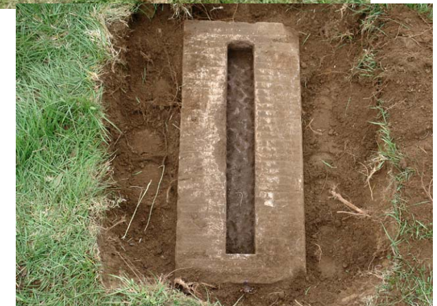
Old base aligned with adjacent markers and reset level.
