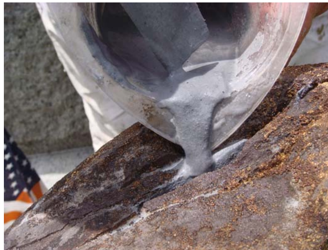
Filling voids with a pigmented flowable grout (VoidSpan PHLc)
