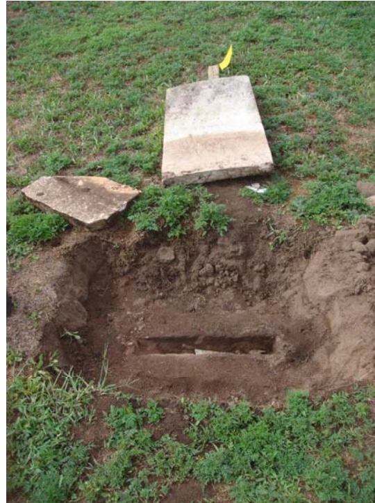
When excavating for resetting often original, or old bases are discovered
