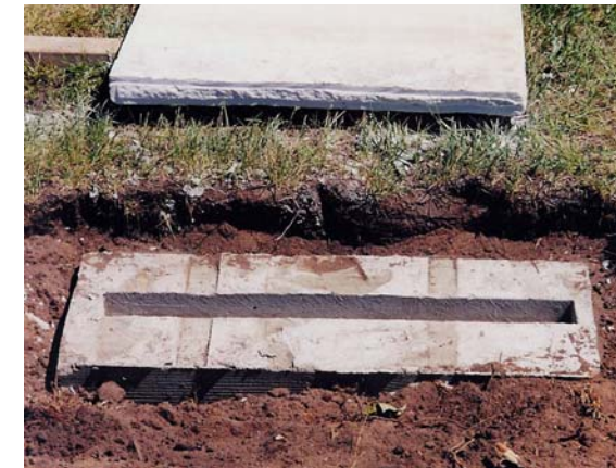
Form removed, ready for resetting marker
