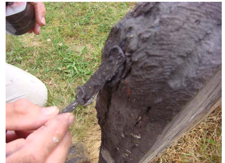
Filling top cavities with a pigmented crack filler by Sto. Excess material will be immediately wiped off with damp sponging
