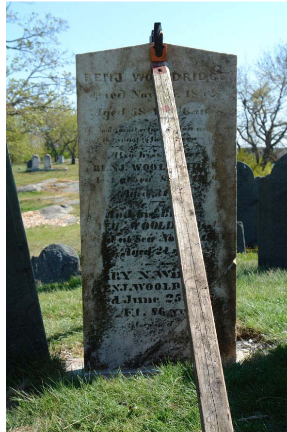
Example of marker reset into slot and braced
