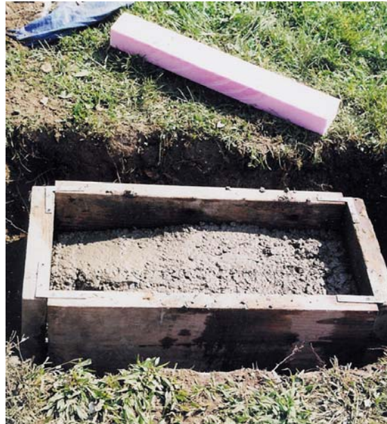
Form for new below grade concrete base
