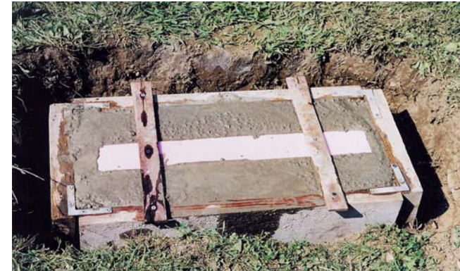
Concrete poured, with form for setting slot in place
