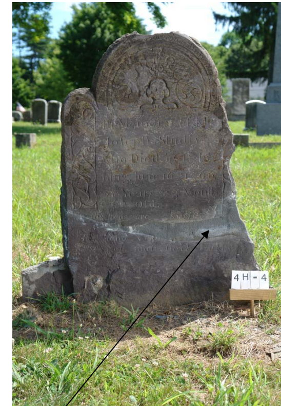
After structural adhesion, losses were filled with Jahn M-70 pigmented mortar.
