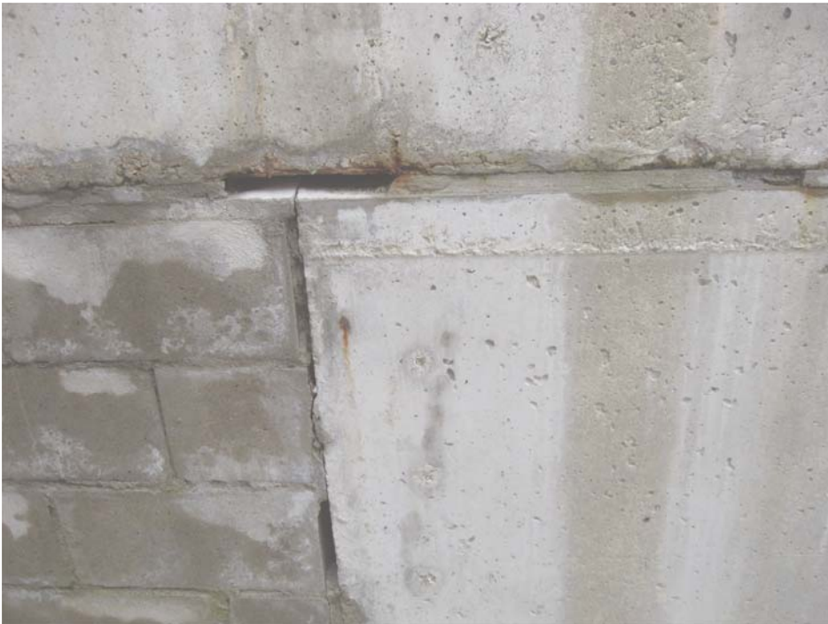
Cracks between block and concrete at steps. This condition was repaired during the summer of 2010 with parging.
