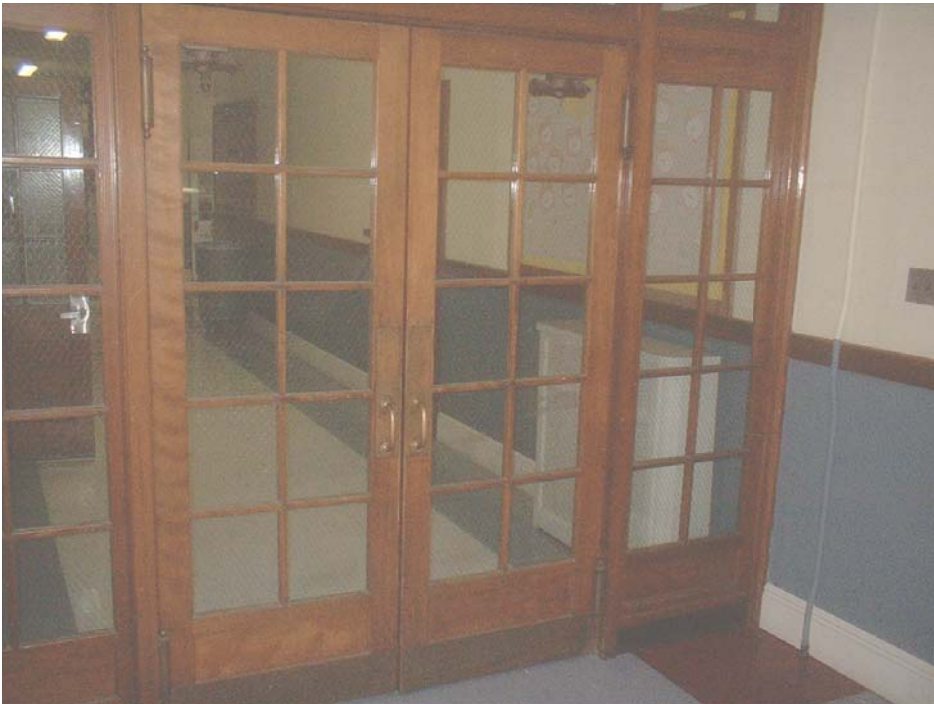
Double 2'-6" doors at stairs; double-acting hinges modified.
