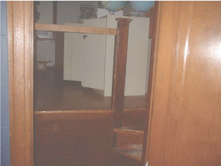
Steps to stage not code compliant.
