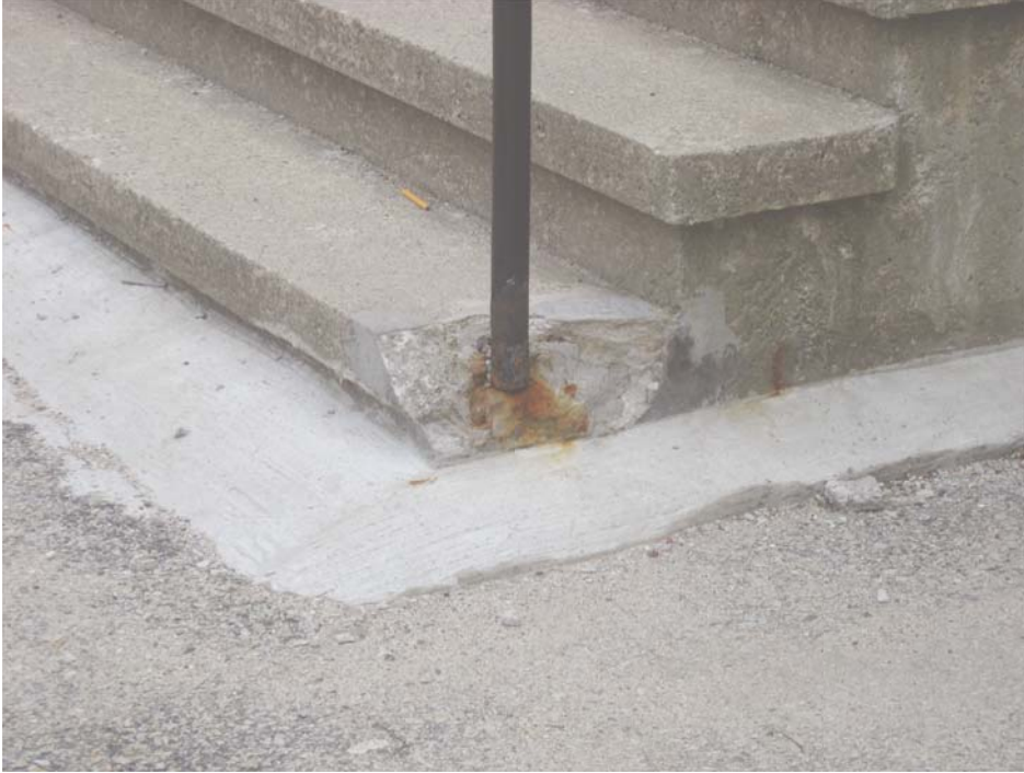
Deteriorating concrete stairs (repaired summer 2010).
