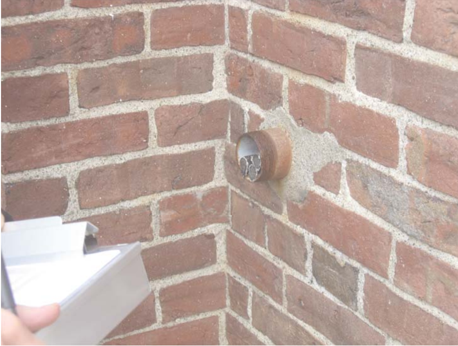
Electrical conduit; large feeder cables inside cut off.
