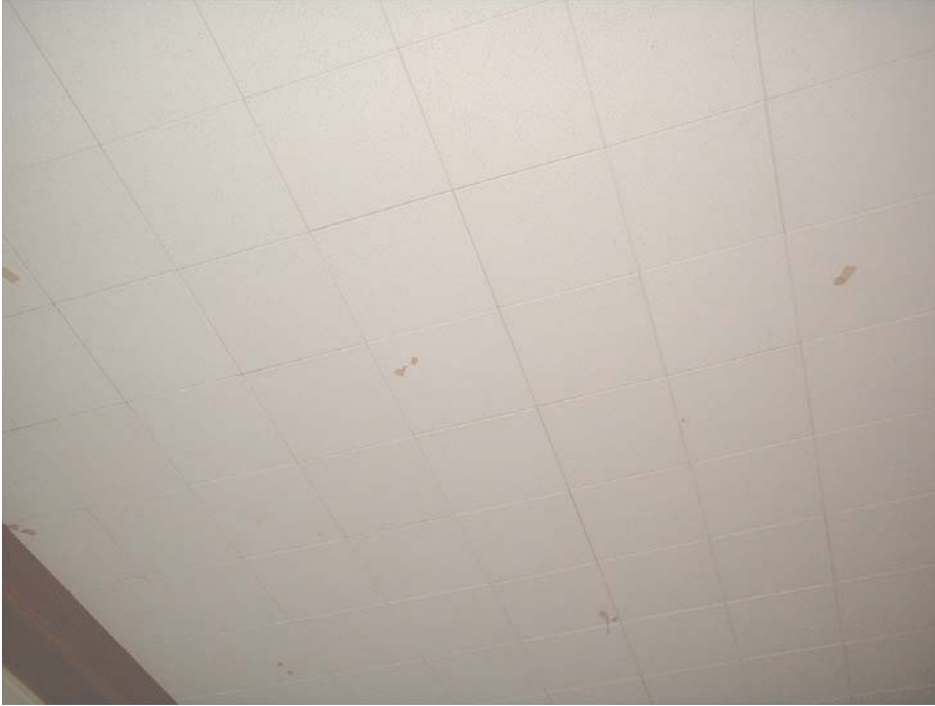
12x12 ceiling tiles reported to have black mastic or black mastic-containing asbestos.
