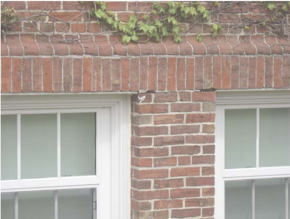
Cracks in brick near windows (lintels).
