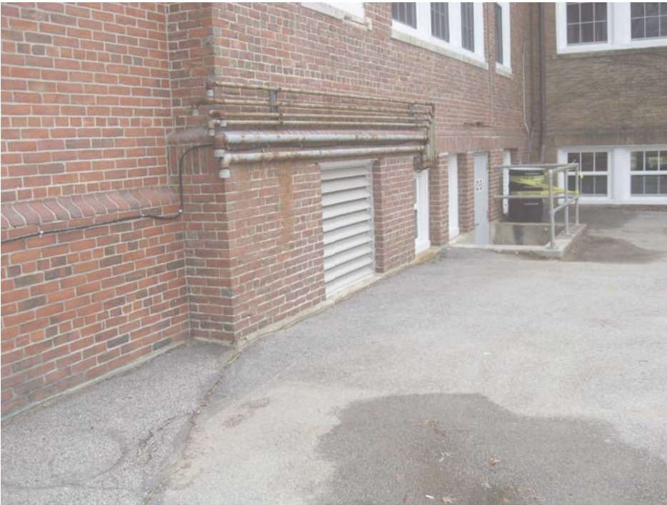
View of stair leading to basement & multiple vent pipes from boiler room.
