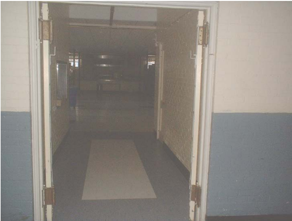
Entrance doors to cafeteria; wood. Narrow doors do not meet access codes.
