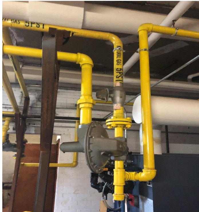
Existing high pressure gas pipe
