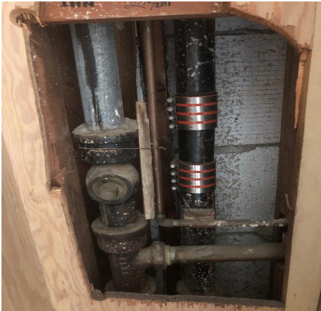
Typical example of original and replacement piping
