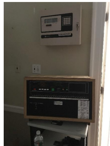
PA Intercom System Head End
