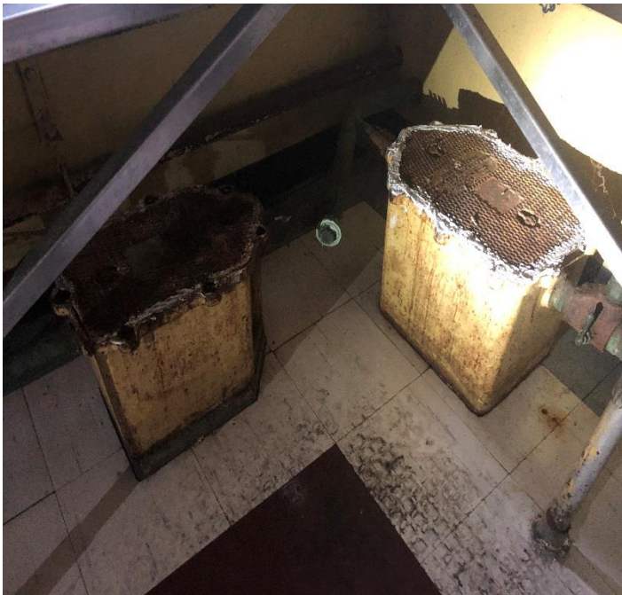
Existing grease interceptors
