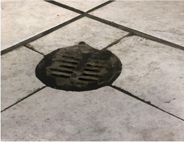
Typical corroded floor drain
