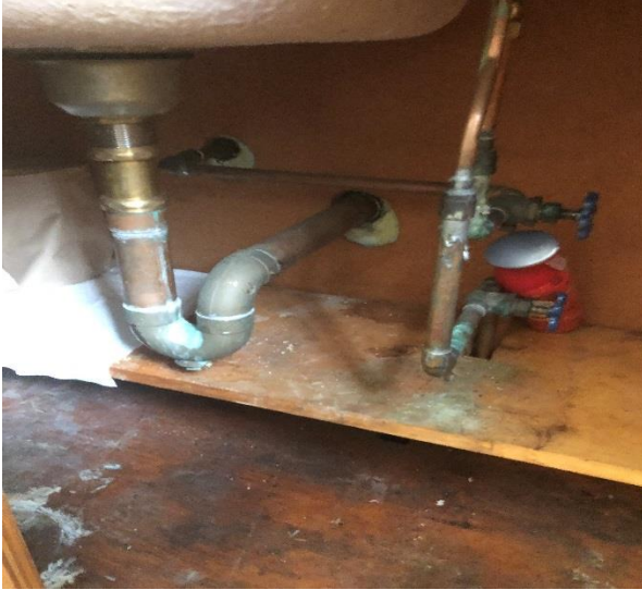
Typical old and corroded fixture piping
