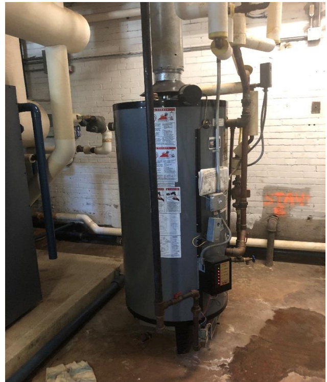
Existing gas fired water heater
