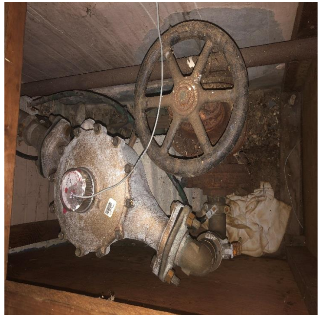
Existing water service and meter
