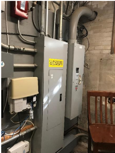
Main Service Disconnect and Main panelboard
