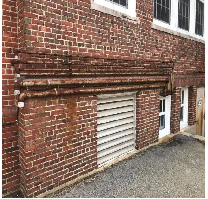
Exterior Gas Vent Piping
