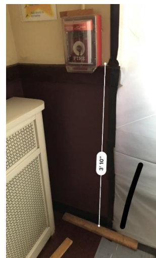
Fire alarm Pull Station Height
