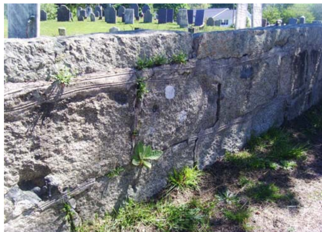
Typical condition of joints
