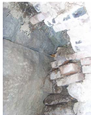
Gap in Front Wall at roof (note missing bricks)
