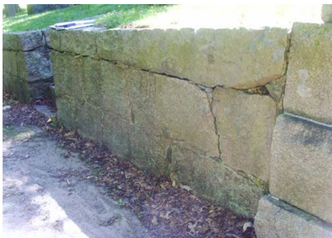
Typical condition of joints
