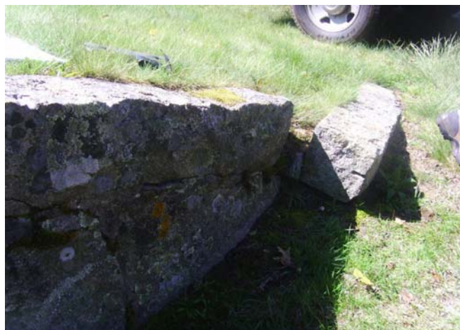
Damaged wingwall
