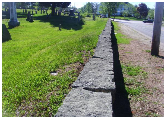
Typical backfill (note rubble backfill)
