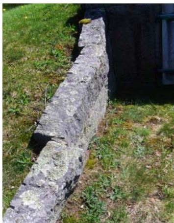
Bulging Wingwall
