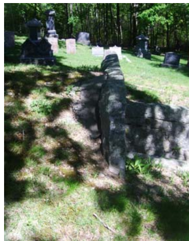
Signs of headwall movement
