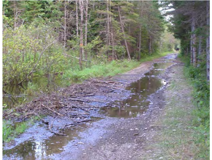
Beaver caused erosion damage, Ashuelot Rail-Trail, NH.
