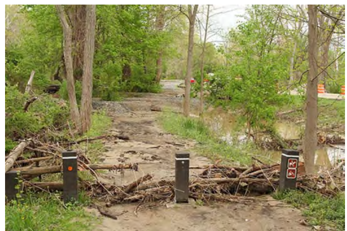
Erosion damage to stone dust trail.
