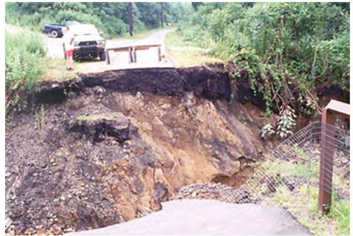
Culvert failure, Allegheny River Trail, PA.
