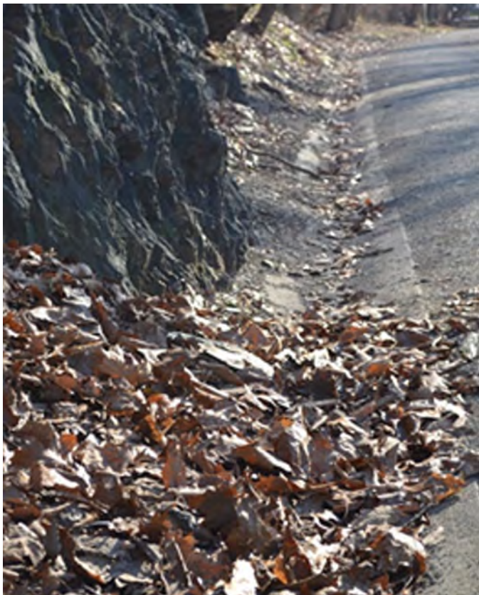
Drainage swale in need of cleaning.
