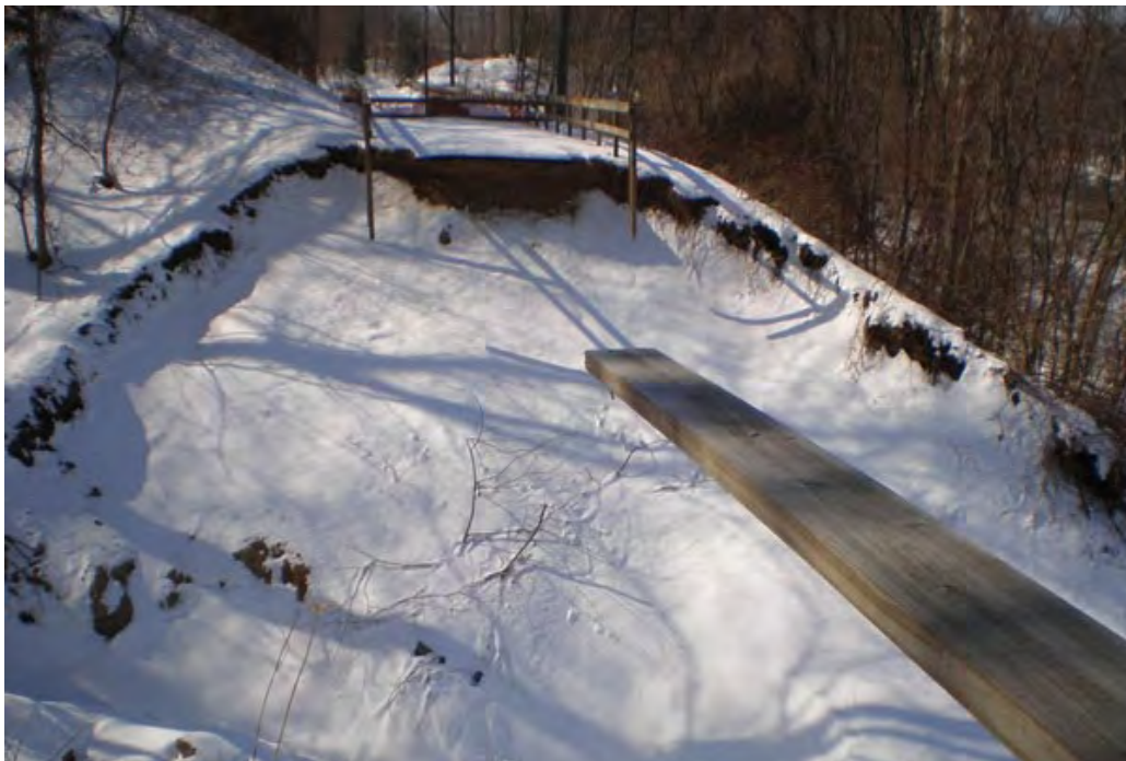
Culvert failure, Manhan Rail Trails, MA.
