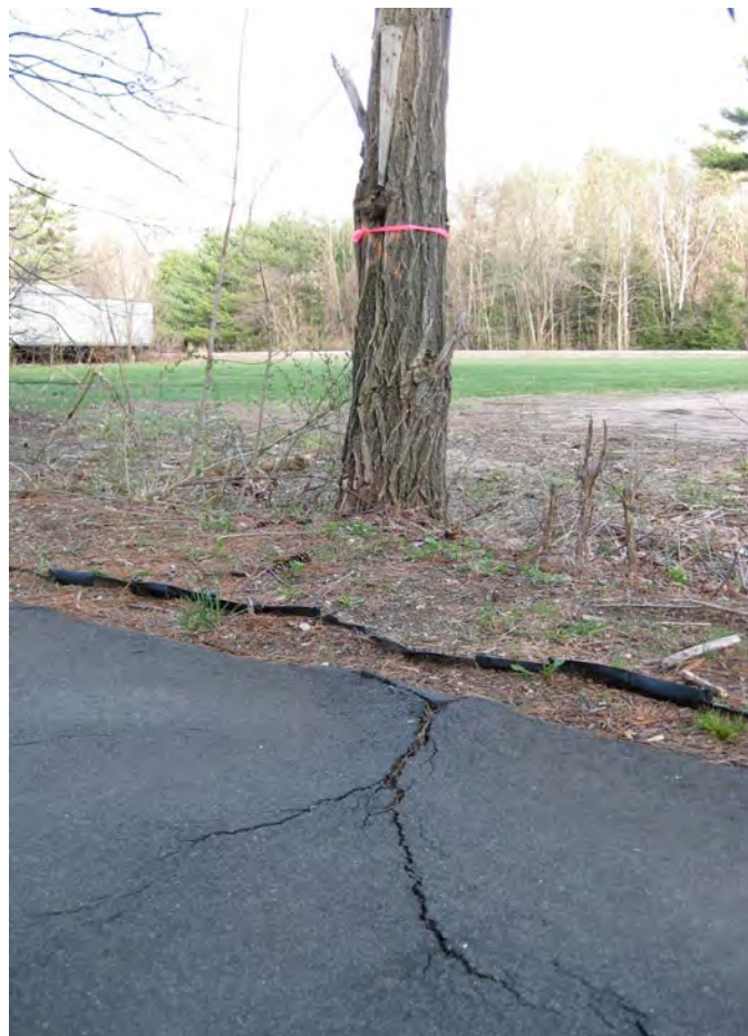
Tree root damage Manhan Rail Trail, MA.
