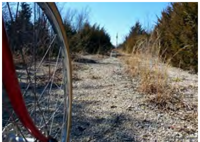
Uncontrolled weed growth through trail surface.
