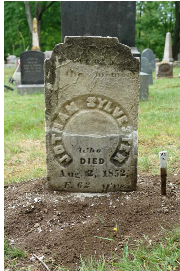
#A3.2 Jotham Sylvester. Open joints filled with Replical crack filler.
