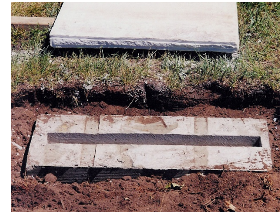
Form removed, ready for resetting marker
