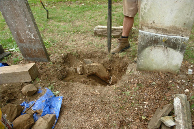
A common cause of tilted markers are roots from nearby trees
