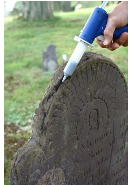
Filling top cavities with a pigmented crack filler by Sto. Material can be applied by trowel or injection. Excess material will be immediately wiped off with damp sponging
