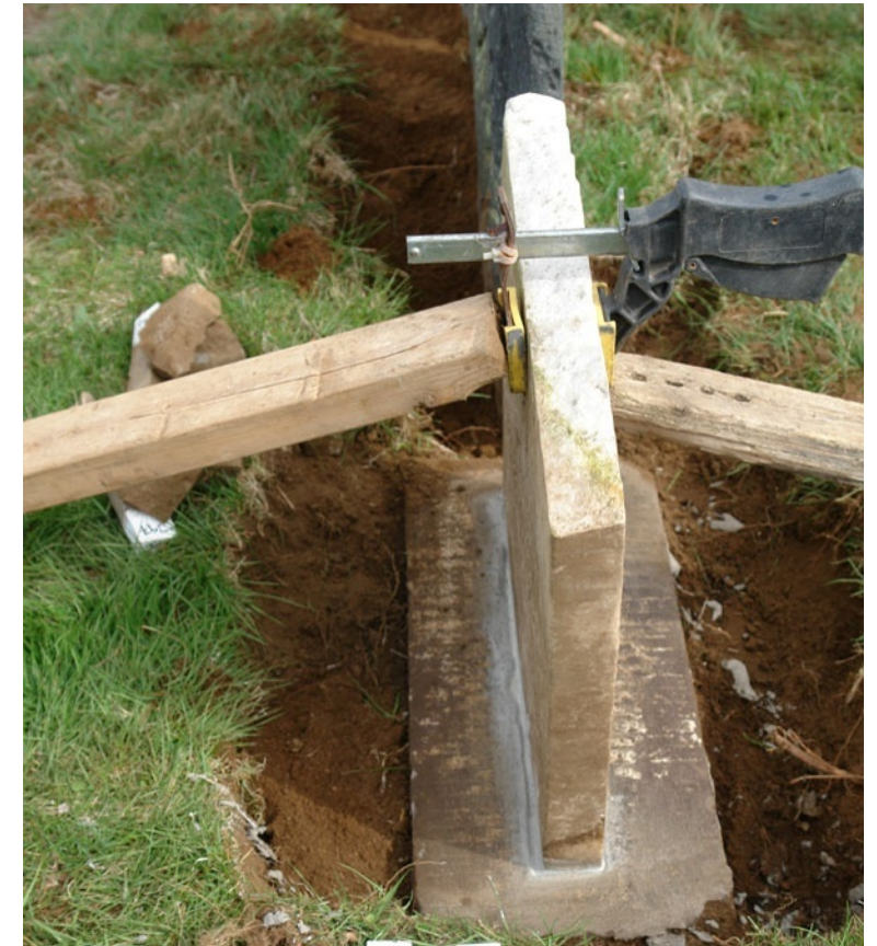
Lower fragment reset into slot and braced. Top fragment will be attached with structural adhesive after grout has sufficiently cured.
