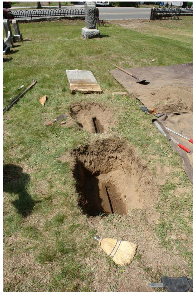
These original bases were raised to an appropriate level and reset plumb
