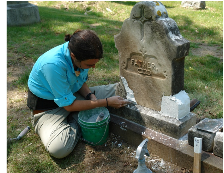
B26.2, William Jacobs. Losses were filled with Jahn M-70 pigmented restoration mortar.
