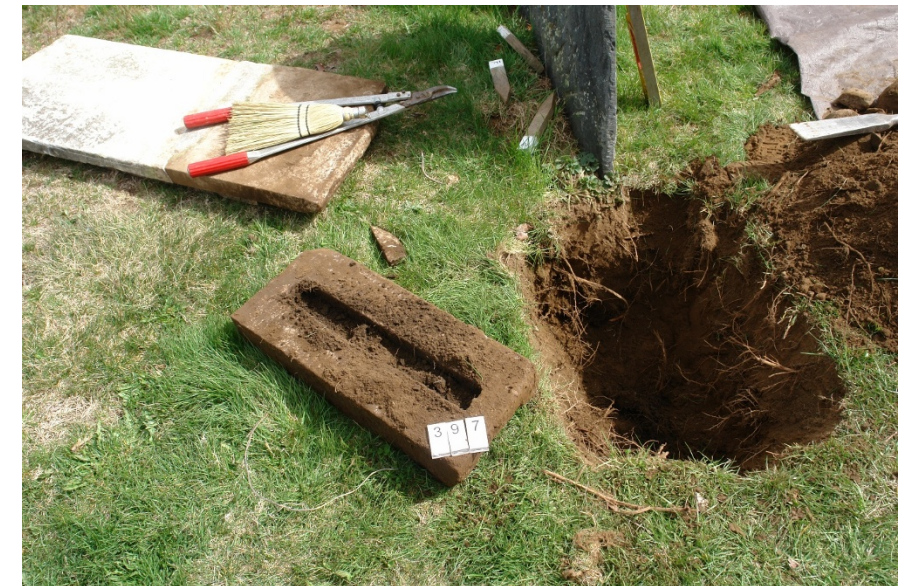
When excavating for resetting often original, or old bases are discovered
