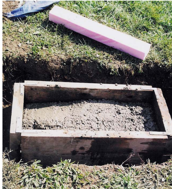
Form for new below grade concrete base
