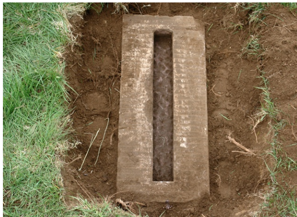
Old base aligned with adjacent markers and reset level.
